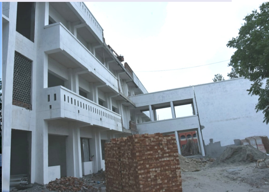
New Girls Hostel Building (Under Construction)
